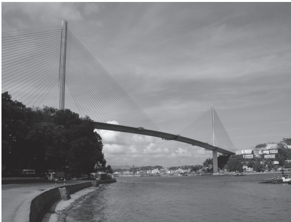
Bai Chay Bridge constructed with ODA of Japan
