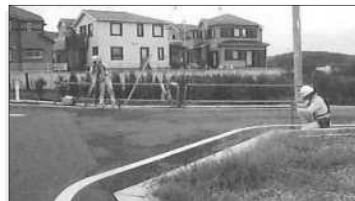
[現況測量の様子]
