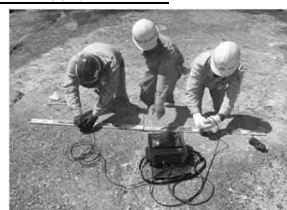
護岸の点検・補修
