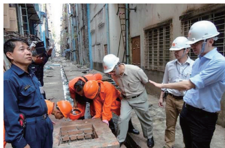
Field survey on sewerage system in Yangon City
