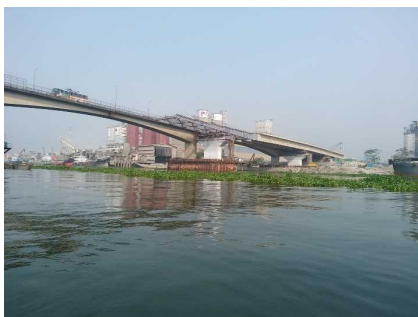
(Photo) The launching erection method (Courtesy of IHI Infrastructure Systems, for the following photos as well)
