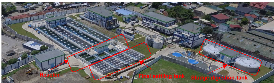
(Photo) Overall view at completion (Courtesy of JFE Engineering)
