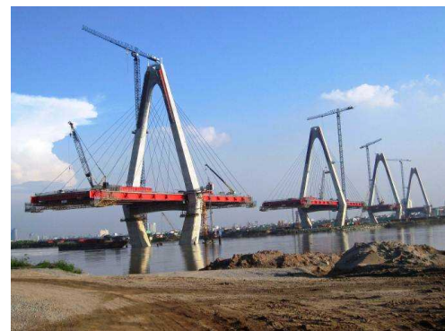
(Photo) Full balancing bridge construction (Courtesy of IHI Infrastructure Systems)
