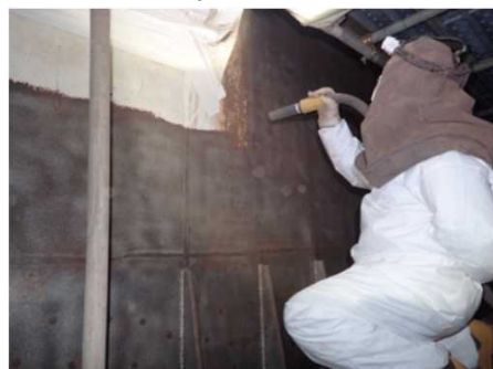
(Photo) The blast method (Courtesy of Obayashi Corporation)
