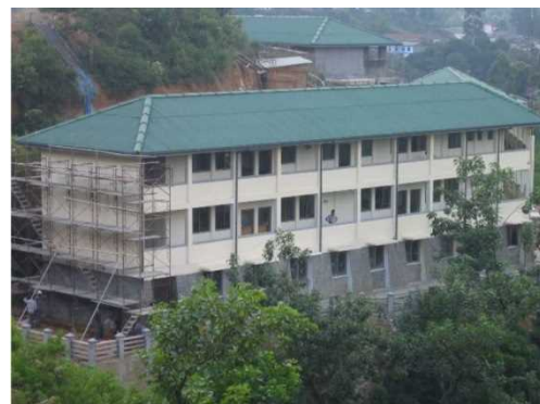
(Photo) Relocated school (Courtesy of Maeda Corporation)
