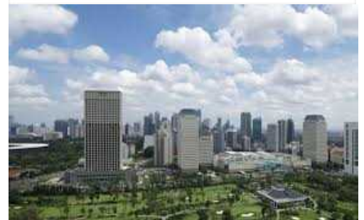
(Photo) Overview of Senayan Square (Courtesy of Kajima Corporation)
