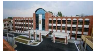
(Photo) Paropakar Maternity Hospital after reconstruction (Courtesy of Hazama Ando Corporation)
