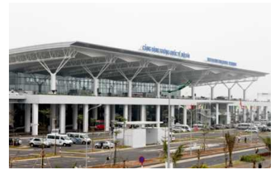
(Photo) Noibai International Airport 2nd Passenger Terminal (Courtesy of Taisei Corporation)
