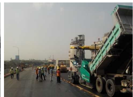
(Photo) PMB paving
