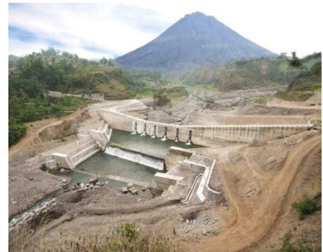
(Photo) Sabo dam (Courtesy of Shimizu Corporation)
