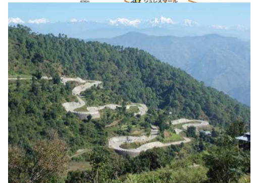
(Photo) Second construction area (Courtesy of Hazama Ando Corporation)
