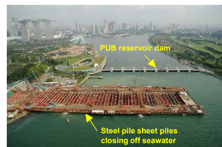
(Photo) The Marina Coastal Expressway Contract 48 construction (Courtesy of Penta-Ocean Construction)
