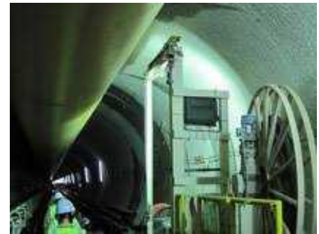
(Photo) Water transfer tunnel
