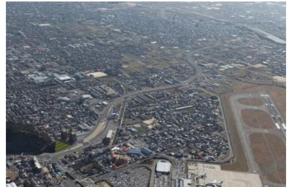
High-standard road connecting airport and city center (Matsuyama Outer Ring Road)
