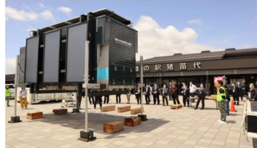
Michi-no-Eki "Inawashiro" (Fukushima Prefecture) Demonstration of "high value-added container" installation
