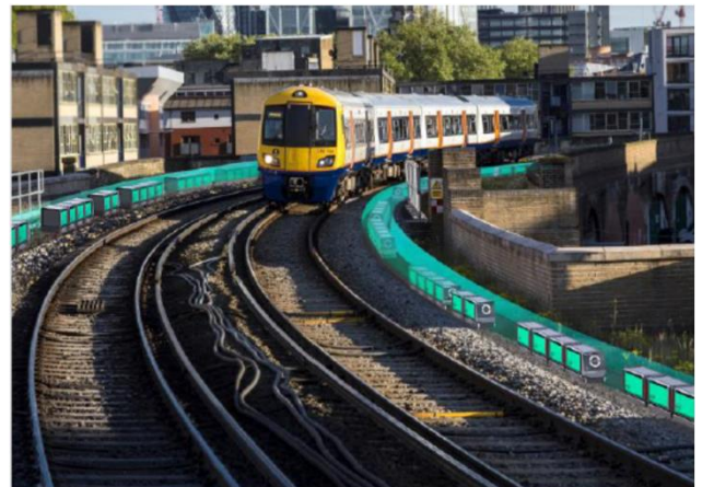
Source: Materials provided by Magway
