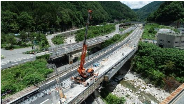
Expressway renewal (Sonohara Bridge, Chuo Expressway)
