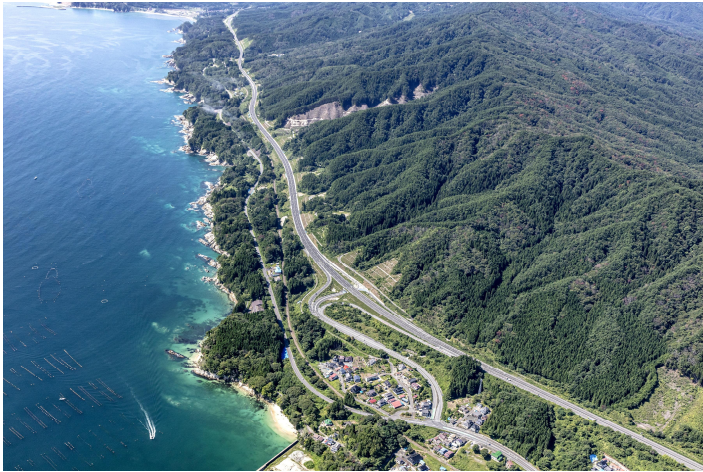
Sanriku Coastal Road (Yamada Town, Iwate Prefecture)
