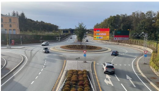
Roundabout (Stavanger, Norway)
